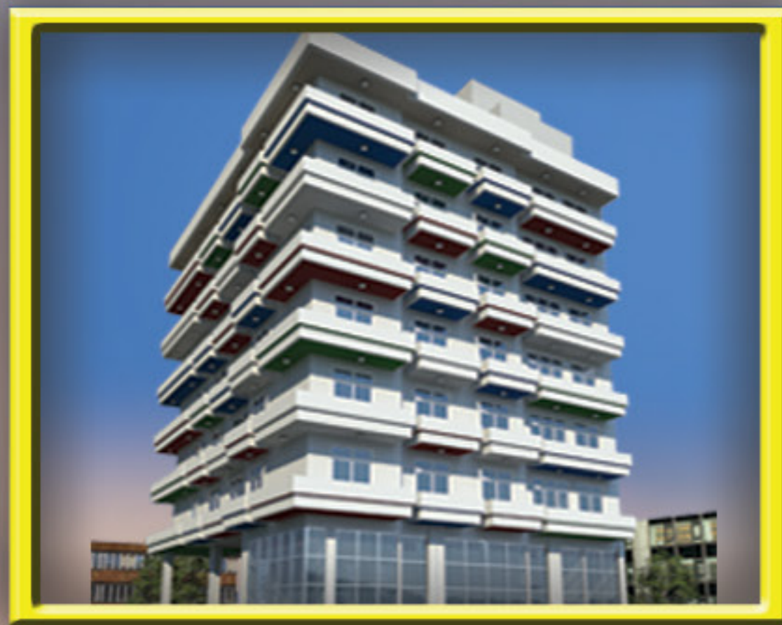
No:45, Peter's Lane, Dehiwala. Ken Tower 05
